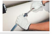
2. Band attaching base to pipeline.
