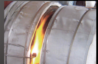
Preheating with torch & ceramic blankets
