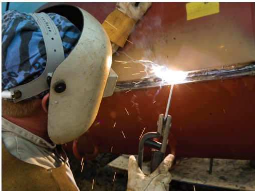
Installation of a TDW tapping fitting
