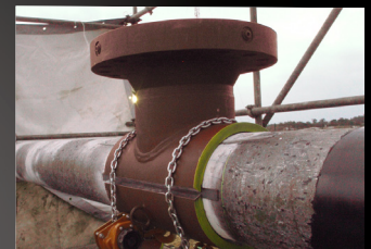
Fit up of welded fitting
