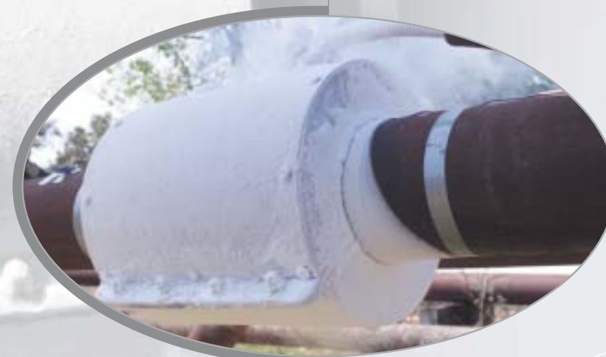
TOP: Technician applies freeze jacket to line. MIDDLE: Freeze temperature reduction is monitored. BOTTOM: Diagonal frost line indicates ice plug is forming. Once freezing is complete, repairs can be made.
