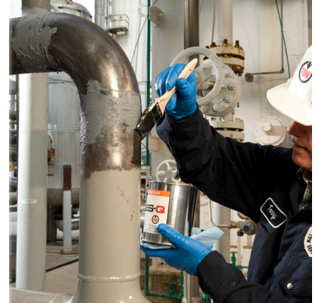
Apply epoxy to surface.
