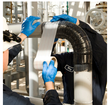
Prepare composite for topcoat.
