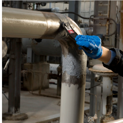
Apply putty to surface.
