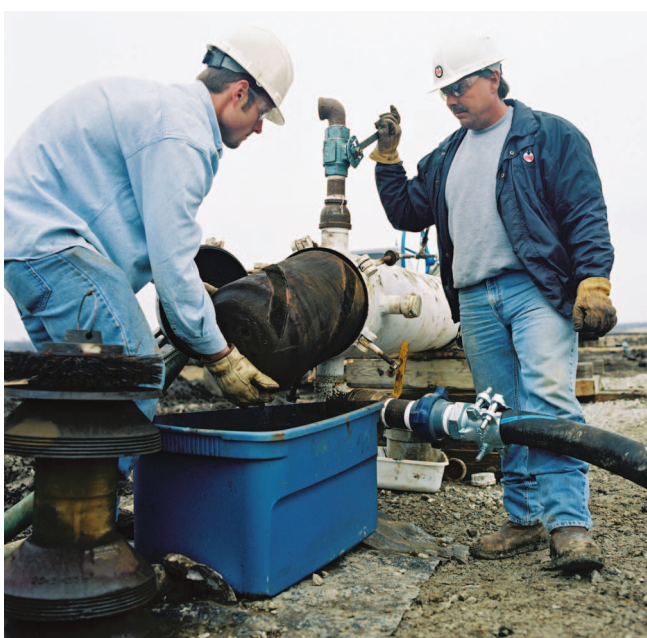
Figure 2. Heavy foam pigs are ideal for pre-cleaning a line because they are forgiving of obstacles and less likely to become stuck.
