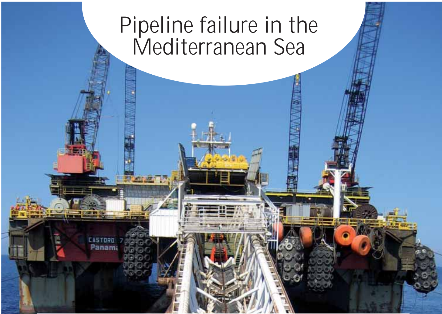
Figure 1. The line has been dewatered and the winch is connected to the PRT, pulling the pipeline onto the vessel.
