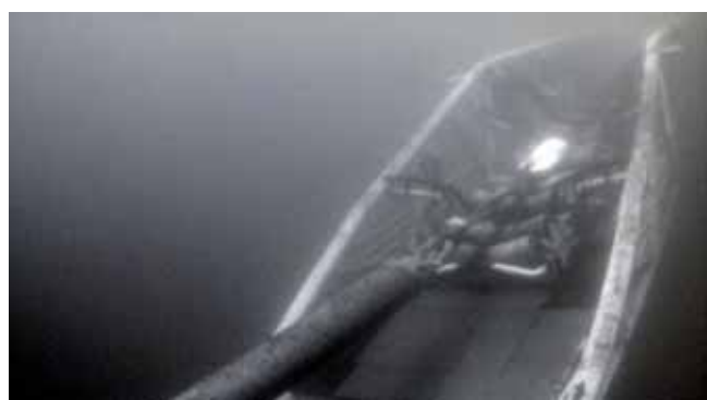
Figure 6. The PRT recovers the pipe by drawing it up the stinger.
