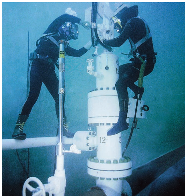
Figure 2. TDW divers carrying out a bypass operation.
