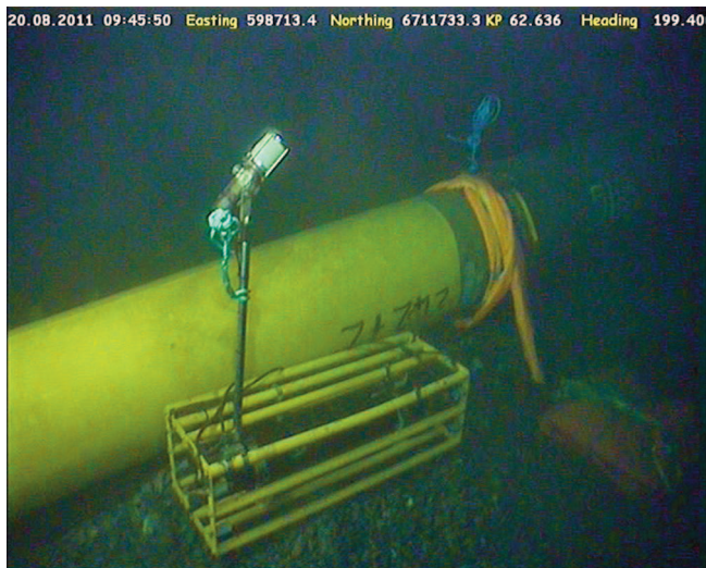
Figure 4. The skid containing the remote logger was placed parallel to the pipeline, close to the subsea pig receiver.
