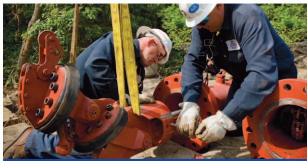
Figure 1. Double block capacity is provided by linking two plugging heads together into a 'train' formation.
